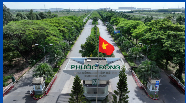
Phuoc Dong Industrial Park - Tay Ninh
