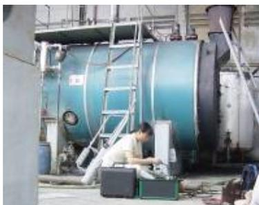
The Vietnam Cleaner Production Centre and its host institution, the Institute for Environmental Science and Technology (INEST), are equipped with portable analytical equipment for both rapid and in-depth assessment of material and energy consumption in various industrial sectors. The portable equipment includes instruments to measure and analyze boiler efficiency, temperature, lighting, motor efficiency, wastewater quality...
