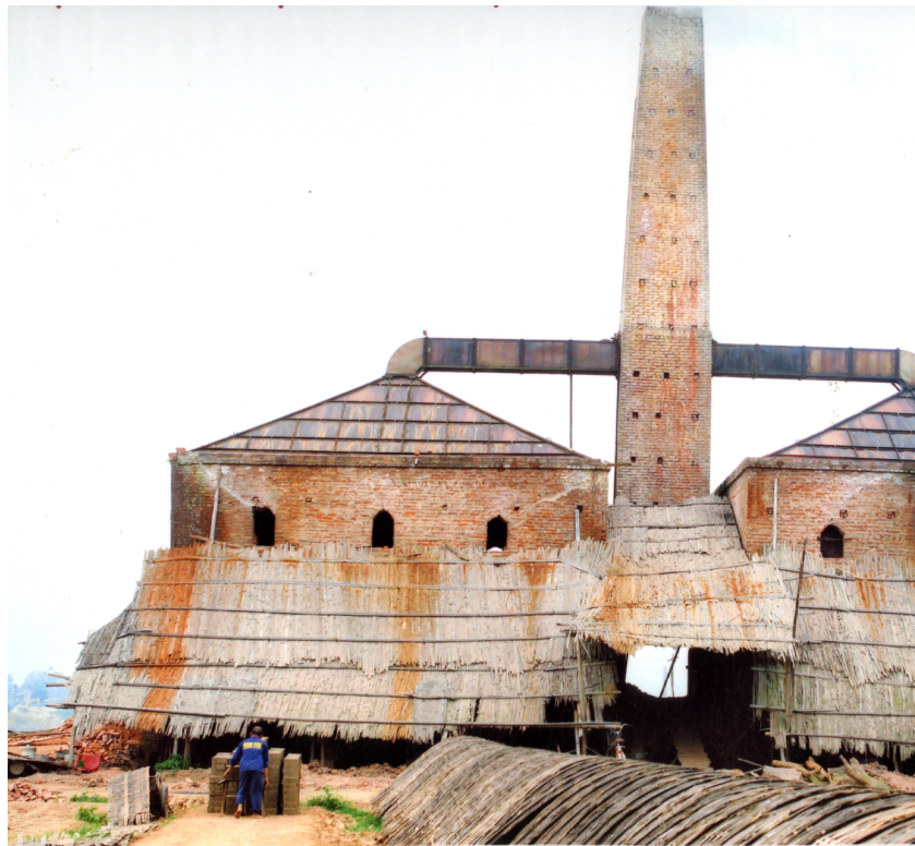
Fired bricks burner
