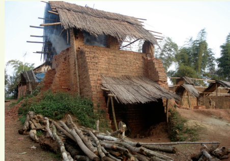
Current traditional brick kiln
