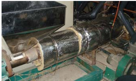
The equipment is now insulated properly
