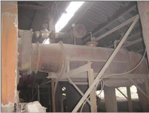
This new economizer in Viet Tri Paper Company brings investment back after 7 months
