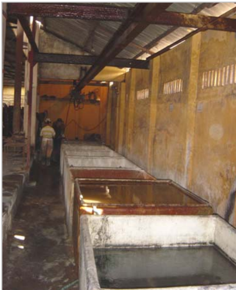
Replacement of manual surface treatment to semi-automatic lines in Truong Thanh Mechanical Company, Nam Dinh (before & after)
